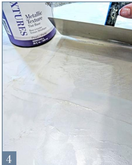
be covered up. Trowel on a random thin to medium thickness of the Cashmere Venetian Plaster mixture. Using the torn edge of a cardboard box, scrape through the plaster where your lines were placed. Now continue to scrape any other designs you would like inside the squares (i.e. swirls, more random lines, etc.). Use sea sponges to make interesting patterns in the plaster areas. Once you have the design all etched out, let dry overnight (*Photo 2*).
